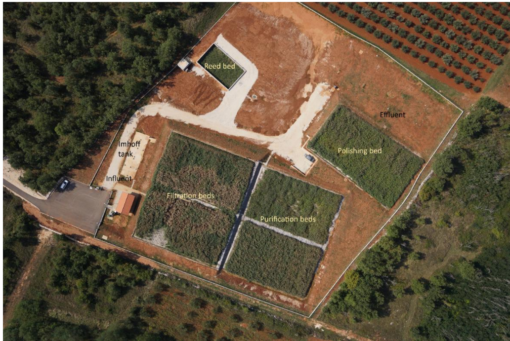
Figure 6: Aerial shot of WWTP Kastelir
