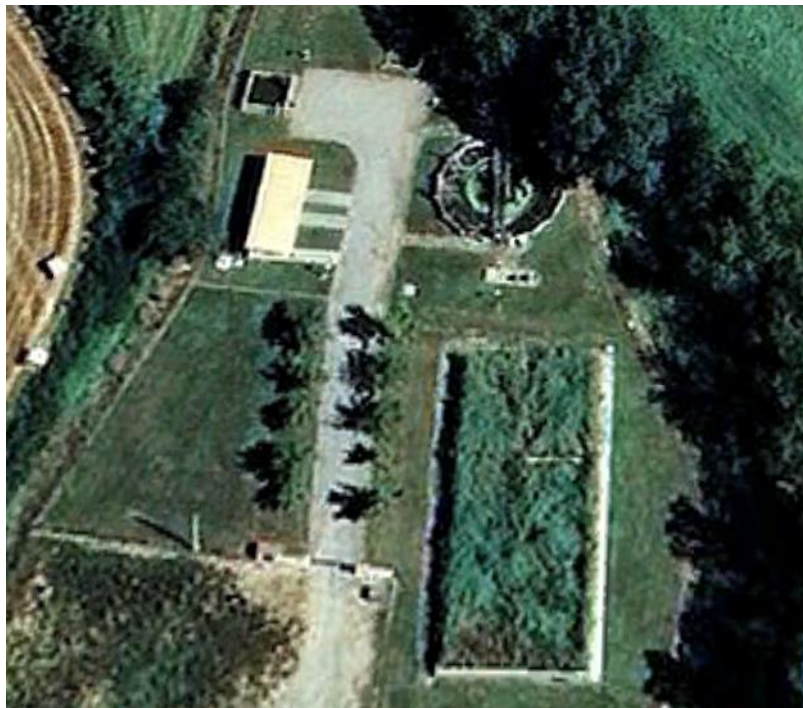
Figure 26: WWTP and reed beds in Sant Boi de Lluçanès 38 .
