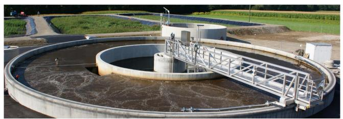
Figure 27: Aeration/anaeration tank and RBs behind in Dellach am Drautal<sup>29</sup>
