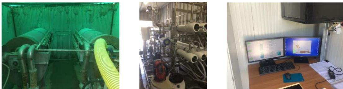
**Figure 3.** View of technological components of the SASA WWTP: primary treatment (centrifuge, left); polishing step (reverse osmosis – RO, centre); remote control (SCADA, right)
