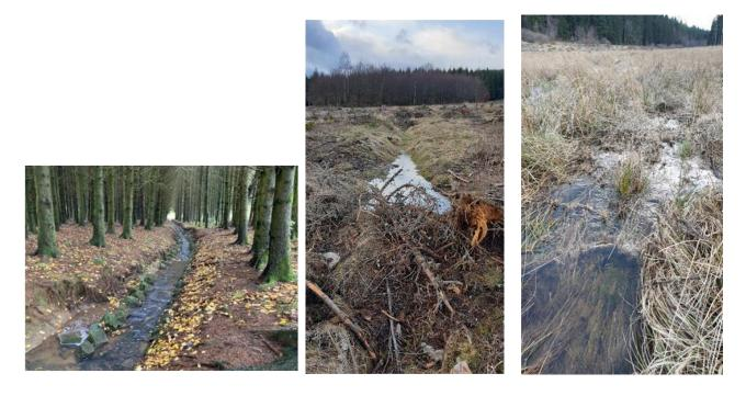
**Figure 30.** Representative snapshots of drainage at three successive stages of restoration of the retention capacity of soils: from left to right, a ditch draining excess runoff as quickly as possible; a blocked ditch, and a wetland originated from the blocking of the drainage.
